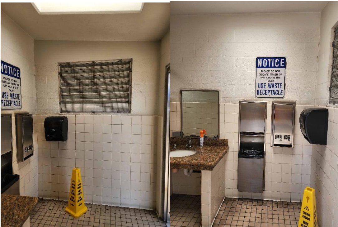
Pier 1 Makai Comfort Station (Women's Restroom) – South Elevation
