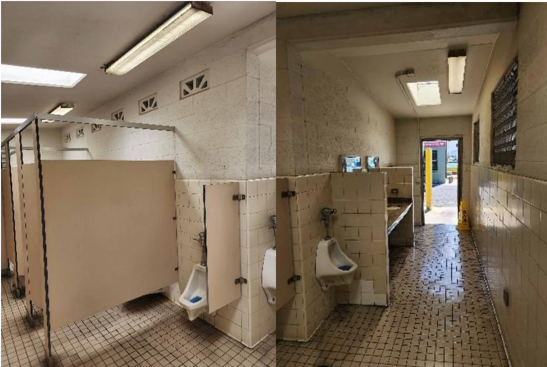
Pier 1 Makai Comfort Station (Men's Restroom) – South Elevation
