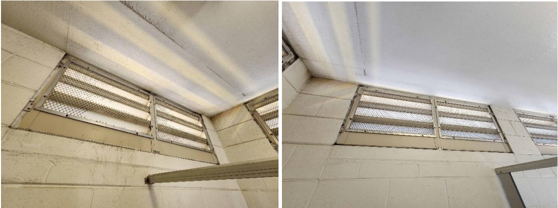
Pier 2 Young Brothers Comfort Station (Women's Restroom) – South West Elevation
