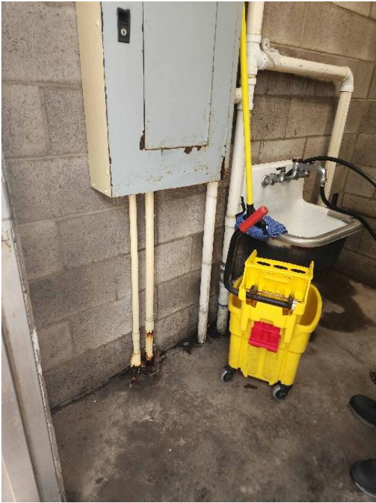
Pier 1 Makai Comfort Station (Janitor Closet) – South Elevation
