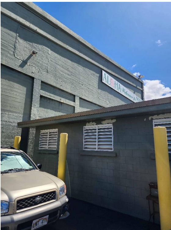
Pier 1 Makai Comfort Station– North East Elevation (Exterior)
