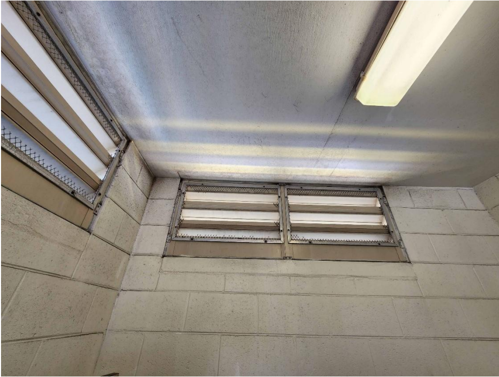
Pier 2 Young Brothers Comfort Station (Men's Restroom) – South East Elevation
