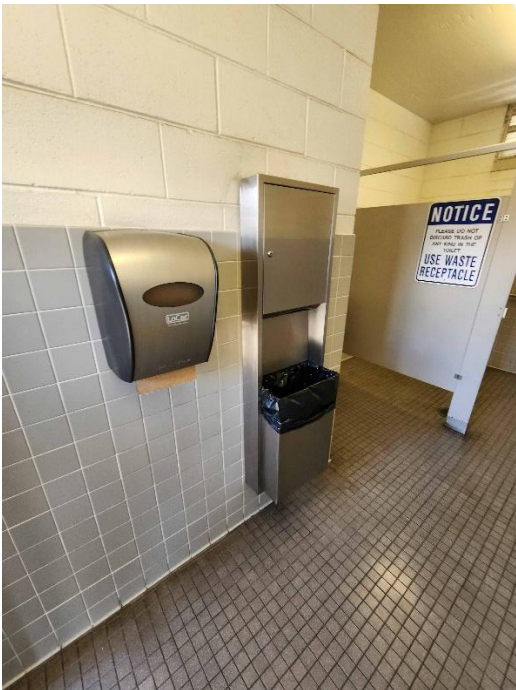
Pier 2 Young Brothers Comfort Station (Women's Restroom) – North Elevation
