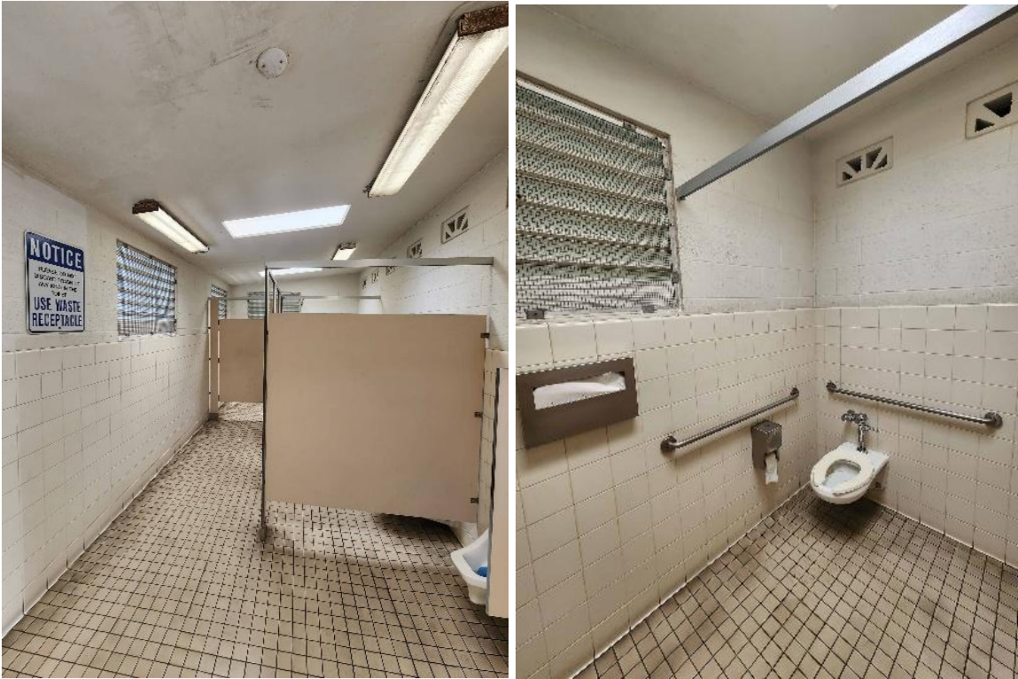
Pier 1 Makai Comfort Station (Men's Restroom) – East Elevation
