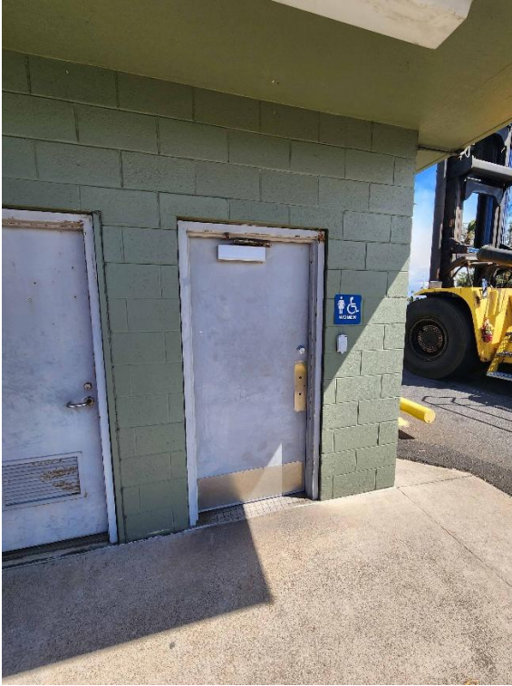
Pier 2 Young Brothers Comfort Station – West Elevation (Exterior)
