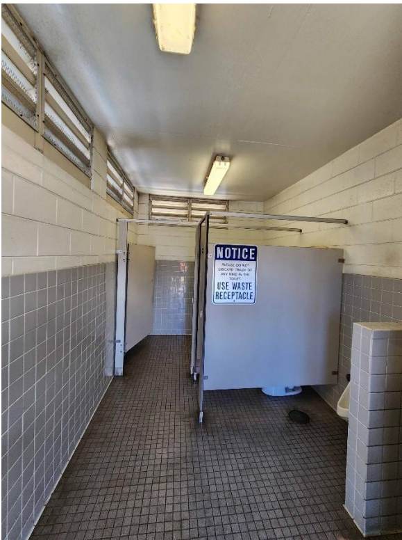
Pier 2 Young Brothers Comfort Station (Men's Restroom) – South East Elevation
