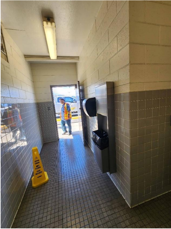
Pier 2 Young Brothers Comfort Station (Women's Restroom) – North West Elevation
